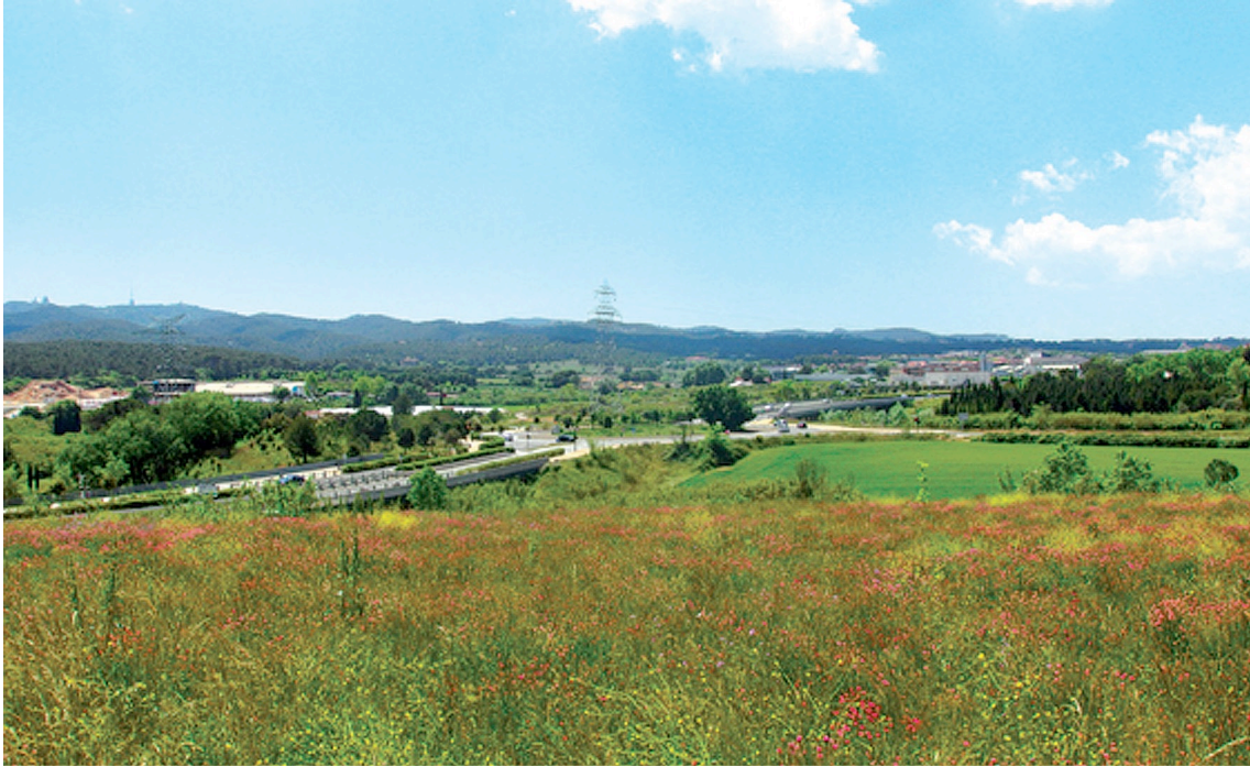
Figure 7. Current state of Airds Catalonia site
