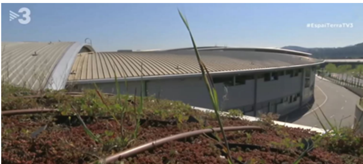
Using nature-based solutions is encouraged in the Alba Park buildings, as is the case with this green roof at the Alba Synchrotron
