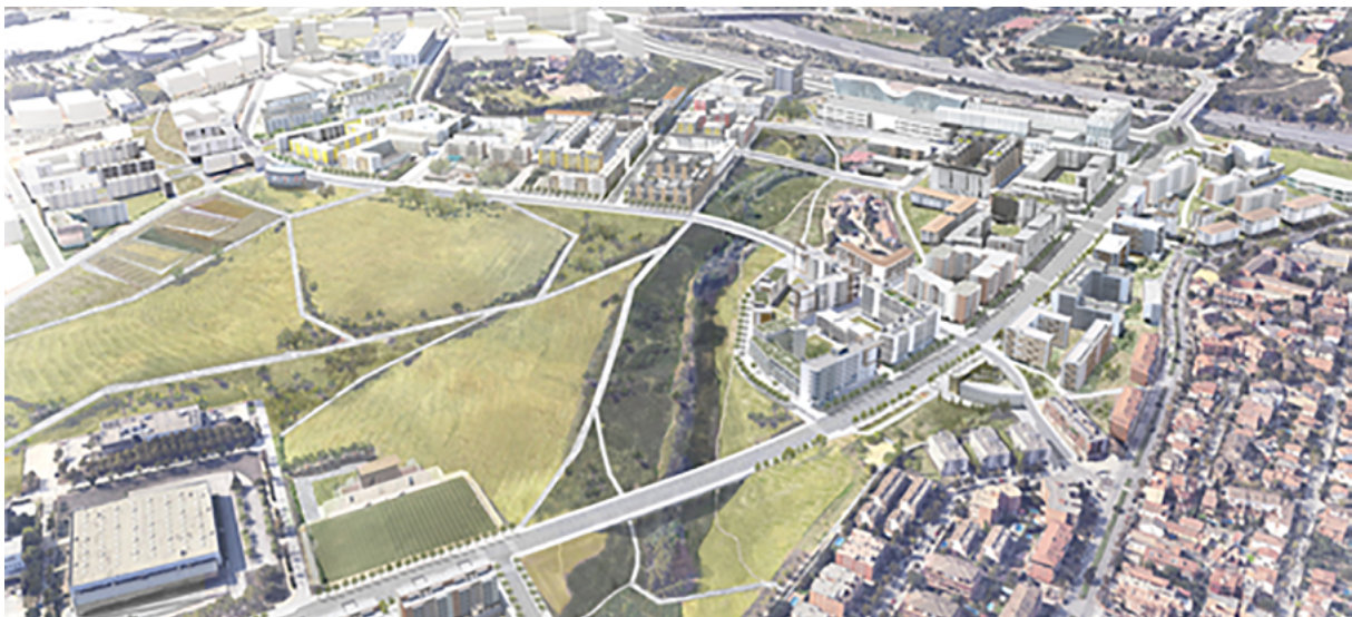
Aerial view of the new residential district in the UDMP interlinked with Cerdanyola
